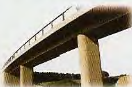
a concrete bridge
